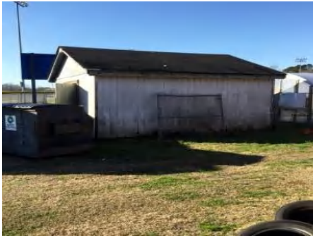
4). North Elevation - Feb 20, 2017
