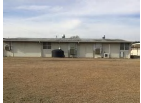
3). Southeast Elevation - Feb 16, 2017
