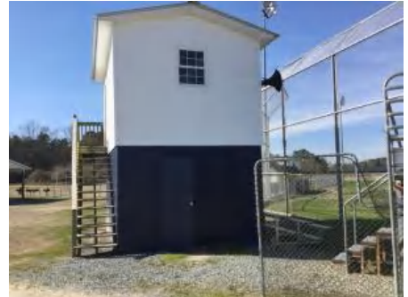
3). Northeast Elevation - Feb 21, 2017
