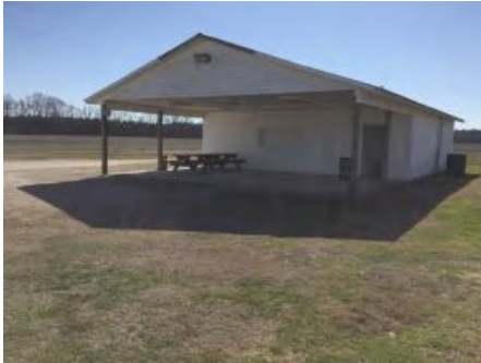
1). North Elevation - Feb 21, 2017
