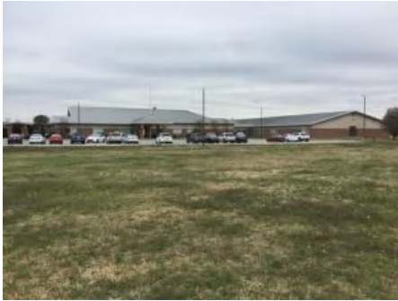
1). Southeast Elevation - Feb 06, 2017
