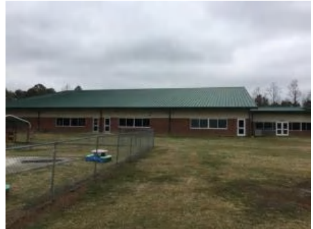
3). Northeast Elevation - Feb 08, 2017
