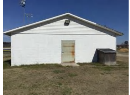
3). South Elevation - Feb 21, 2017
