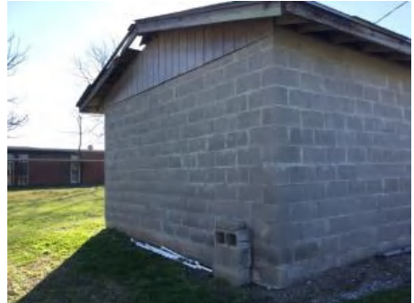
3). North Elevation - Feb 20, 2017
