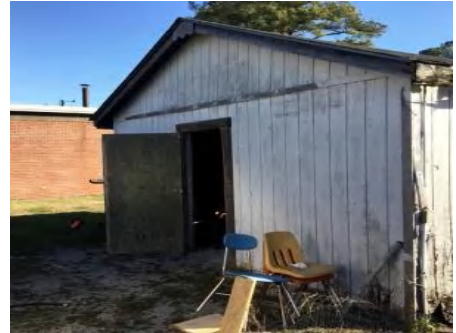
3). East Elevation - Feb 20, 2017
