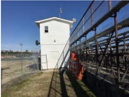
1). South Elevation - Feb 21, 2017
