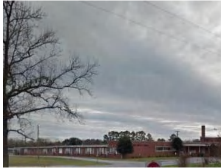
2). Northeast Elevation - Feb 16, 2017
