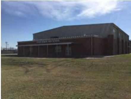
1). North Elevation - Feb 21, 2017
