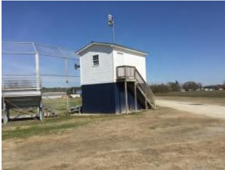
1). Southeast Elevation - Feb 21, 2017
