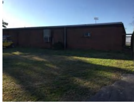
2). North Elevation - Feb 20, 2017
