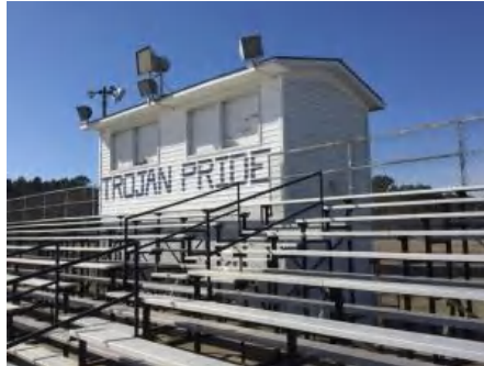
2). East Elevation - Feb 21, 2017
