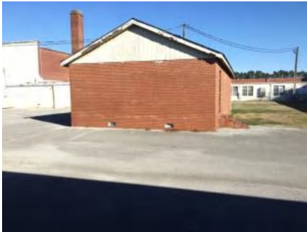
4). South Elevation - Feb 20, 2017
