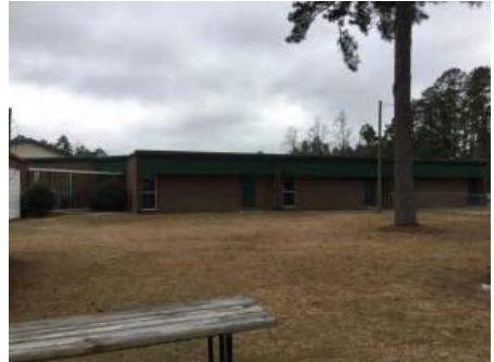
3). North Elevation - Feb 08, 2017
