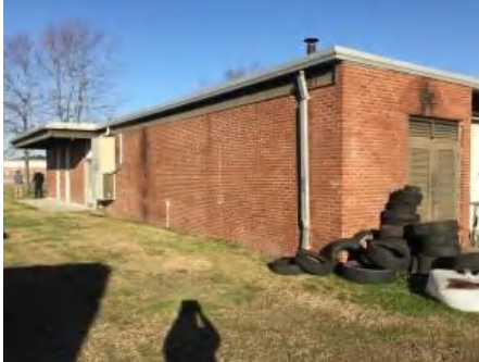
4). South Elevation - Feb 20, 2017
