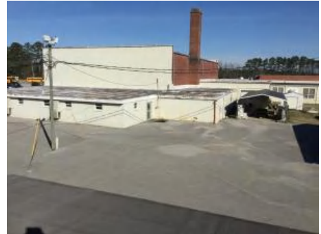
3). Partial South Elevation - Feb 20, 2017
