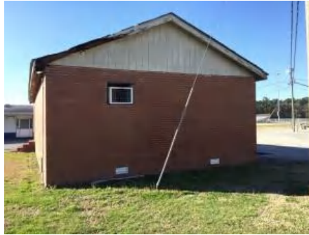
2). North Elevation - Feb 20, 2017
