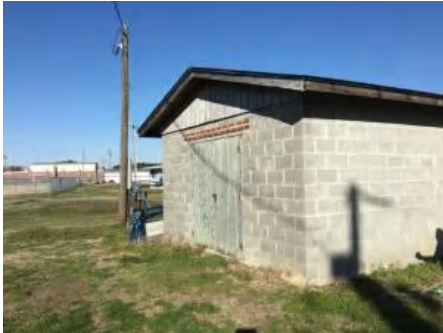
1). South Elevation - Feb 20, 2017
