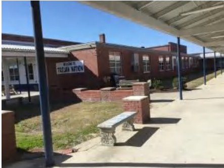
1). North Elevation - Feb 20, 2017
