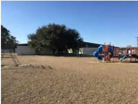
4). Southeast Elevation - Feb 21, 2017
