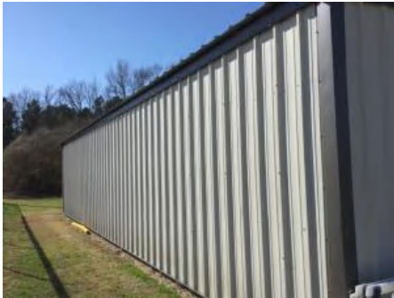
4). Southeast Elevation - Feb 21, 2017
