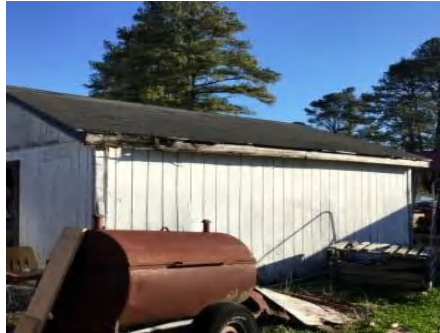
2). South Elevation - Feb 20, 2017
