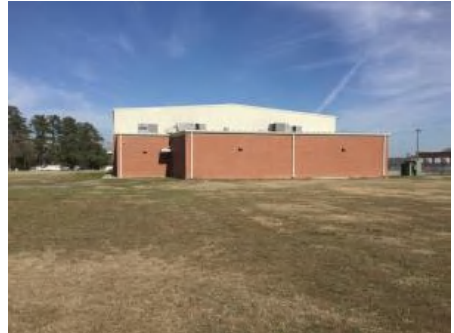
3). South Elevation - Feb 21, 2017
