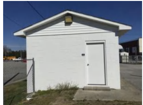
3). South Elevation - Feb 20, 2017
