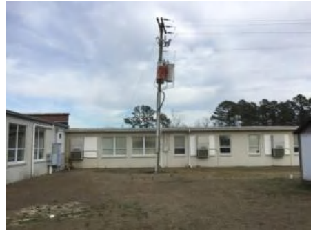
3). Southeast Elevation - Feb 16, 2017
