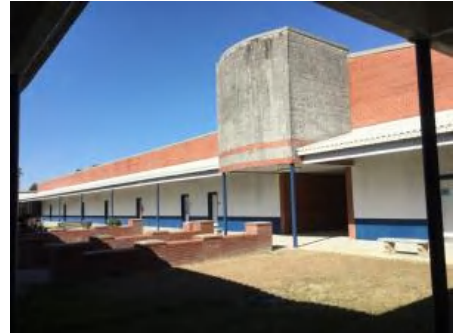
3). South Elevation - Feb 20, 2017
