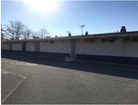
1). North Elevation - Feb 20, 2017
