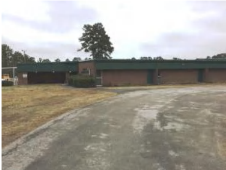
1). South Elevation - Feb 08, 2017
