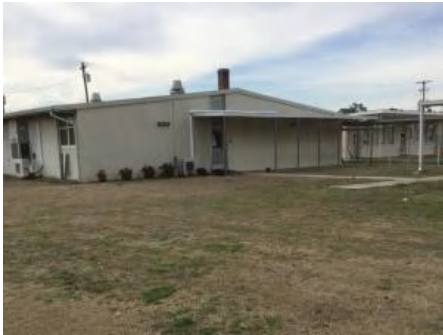
4). Northeast Elevation - Feb 16, 2017
