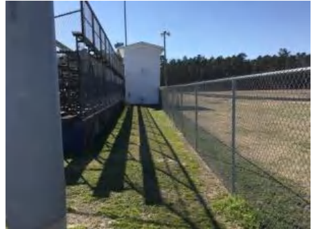
3). North Elevation - Feb 21, 2017
