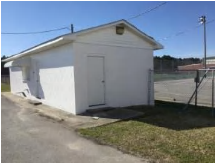
1). North Elevation - Feb 20, 2017
