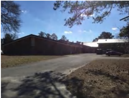
4). Northeast Elevation - Feb 15, 2017
