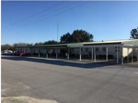
1). Northeast Elevation - Feb 21, 2017
