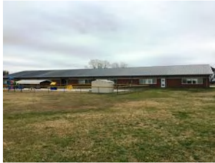
2). Northeast Elevation - Feb 06, 2017
