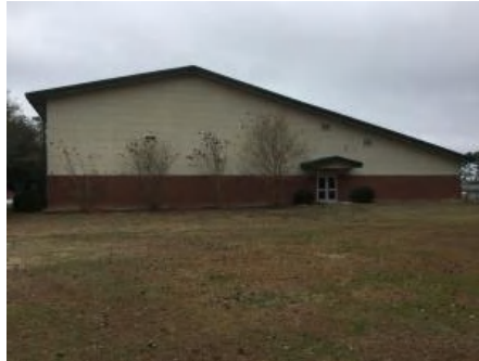
2). Southeast Elevation - Feb 08, 2017
