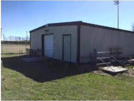
1). Northeast Elevation - Feb 21, 2017
