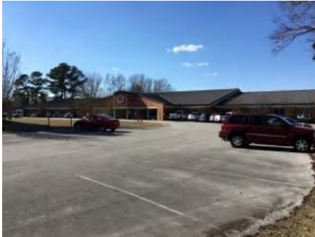
1). Southeast Elevation - Feb 15, 2017
