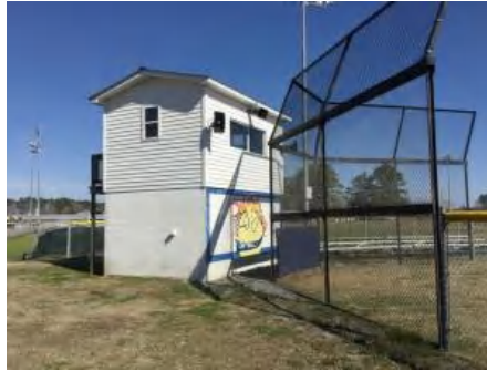
2). Southeast Elevations - Feb 21, 2017
